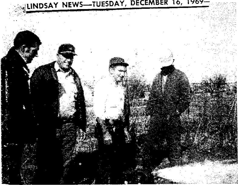
WATER FLOWS from a fire hydrant in Bradley as final inspection of the new water system is made. From the left are Gale Andrews, FHA Grady county supervisor; Carl Stephenson,, board member; Fred Dennis, board chairman and Fritz Badertscher, board secretary.
